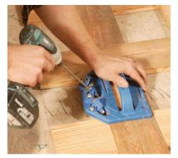
Fasten the grid to the subfloor. The author used a decking jig to locate concealed pocket screws in the board edges. Perimeter ends were fastened with two surface-mounted holes that were then plugged.
