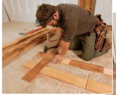
**Pick a corner and start there.** Begin the weave by interlocking two boards at one corner. After applying glue to the dado facing up, push the joint together, using a dead-blow hammer to help with tight joints.
