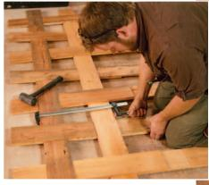
A one-man weave. Run all the horizontal boards from the first vertical, then work in the next vertical. Bar clamps, and later the hammer, help to overcome the resistance of the weave, especially towards the end as the tension increases.
