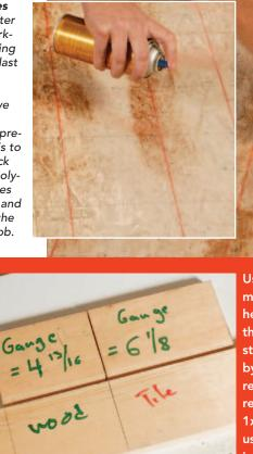
Using a story pole for layout isn't the most original idea, but in this instance it helped me make an accurate layout on the floor and mark the dadoes on the stock in the exact same position. I started by cutting two gauge blocks, one to represent the width of the wood and one to represent the slate. The story pole was a 1x4 on which I marked a centerline. I then used the gauge blocks to lay out alternating wood and slate spaces. Different colored ink differentiated the two.
