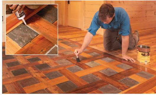
**Finishes need to be forgiving.** The author used a sanded acrylic caulk by Laticrete (inset) as a flexible buffer between the seasonally mobile wood and the immobile slate. After laying down a careful 1/8-in. bead, he smoothed the bead with a wet finger, then used a damp rag to clean up the excess. The wood was sealed with several coats of Waterlox.
