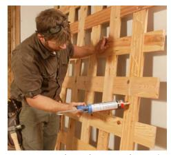
It's easy to work on when vertical. A rigid assembly will lean nicely against the wall. Apply construction adhesive to the back sides of the grid members, then lay the grid back down into place.
