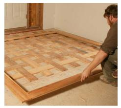
**Make the frame and drop it on.** For the grid's joints to be as tight as possible, trim the grid to the chalklines, take careful measurements, and assemble the frame with pocket screws in the shop.
